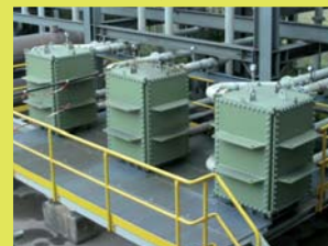
3 HEATEX® HXE75 – 180m 2 – Wash oil cooler on coke oven gas BTX removal plant – Germany
