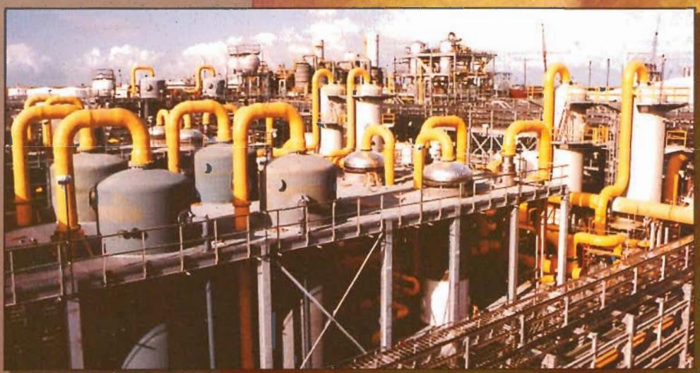
GR-KOR® (FRP) pipe spools connected to Chlorine Drying Towers
